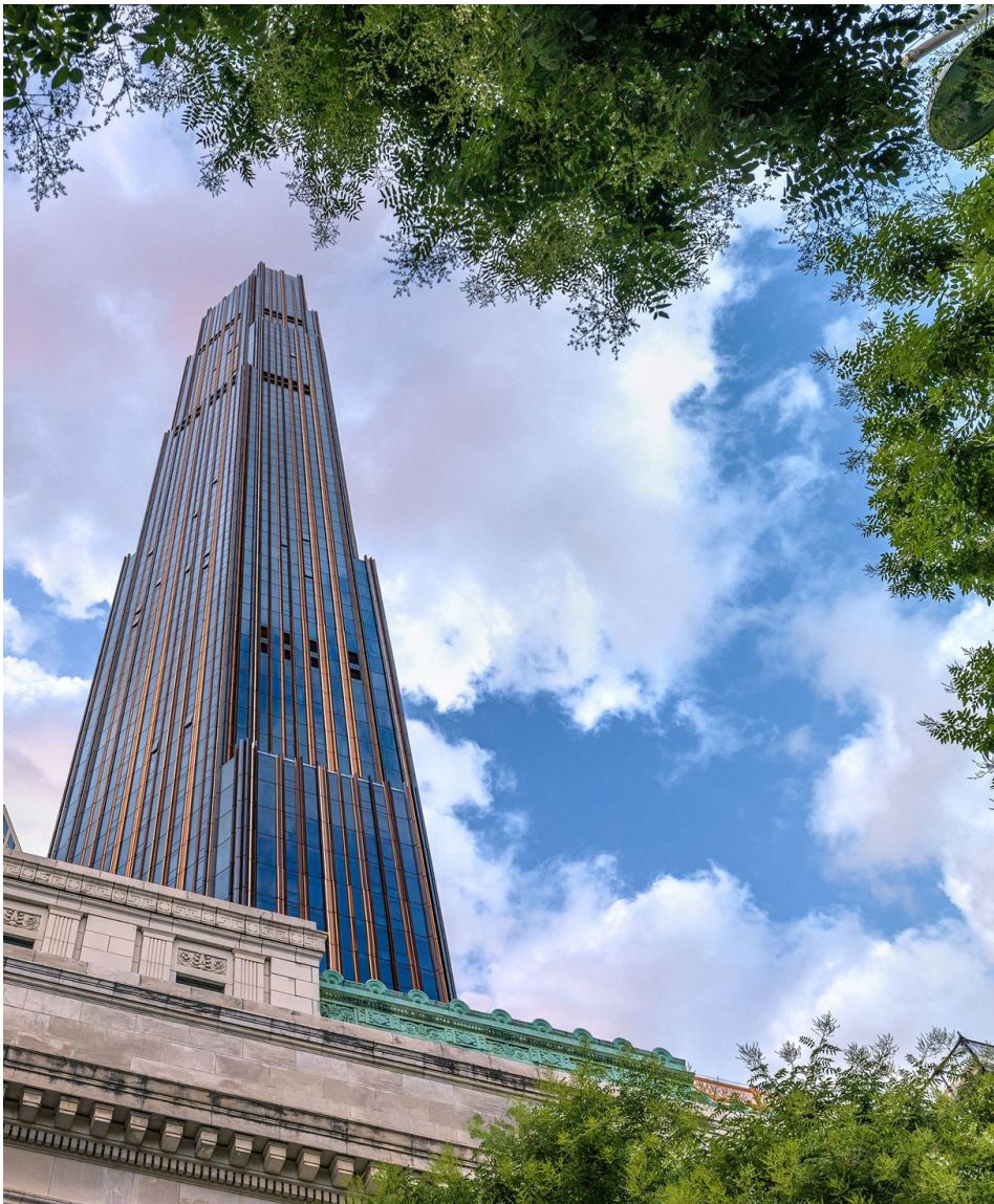
View up from the Entrance to the Brooklyn Dime Savings Bank
