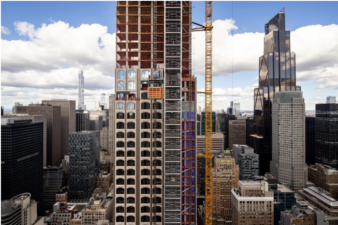
Exterior Photo of the Construction Progress
